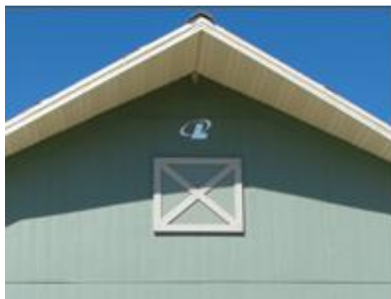
*Overhangs with steel soffit & fascia
