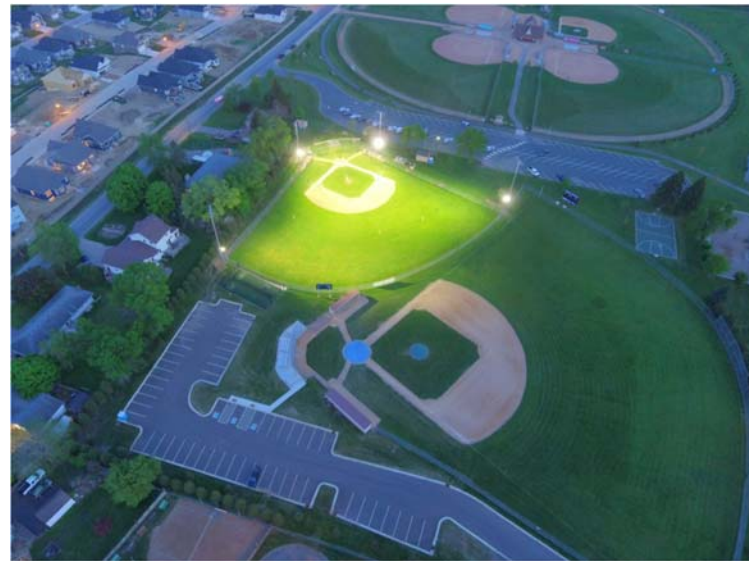
Above: New Musco LED Total Light Control fixtures lighting up the Little League Field in Hamel Legion Park on May 17, 2018 with no light spilling onto nearby properties.
