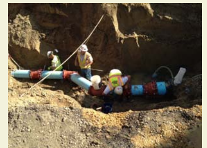
Replacement of a section of Water Main along Tower Drive and Hamel Road.
