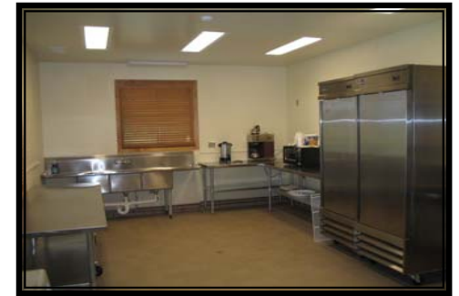
The facility's service area includes a service window with a retractable stainless steel door, stainless steel counters, sink area, refrigerator/freezer, microwave, coffee maker, and a rear entrance.
