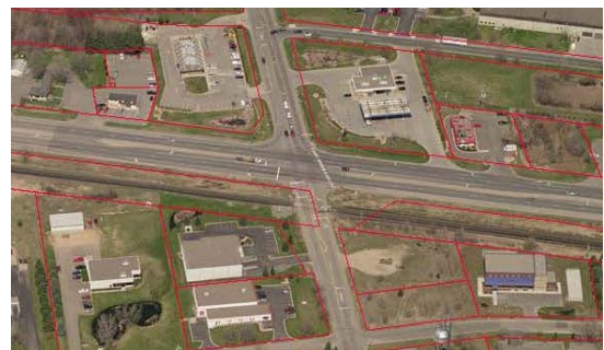
Current Highway 55 at County Road 116/115 Intersection
